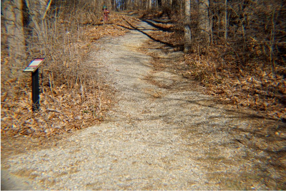
Figure R.1 Significant erosion where trail exits the very southern end of "Stadium Woods"
