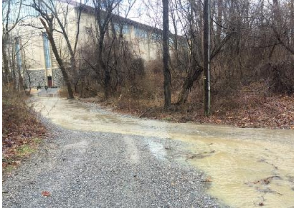
Figure 2.5 Water running down the emergency ingress/egress access road in Virginia Tech's "Stadium Woods" during heavy rain event (road is built on an ephemeral stream). The new indoor athletic practice facility can be seen in the background, 2/24/2016.
