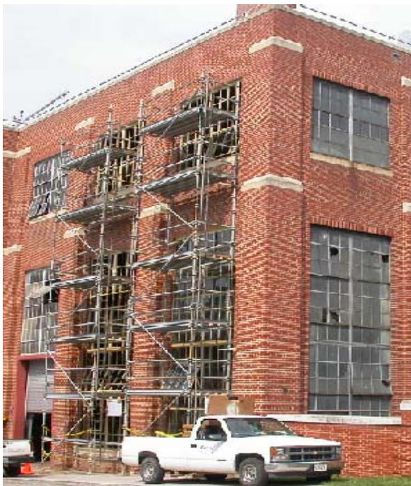
Power Plant Windows Restoration
