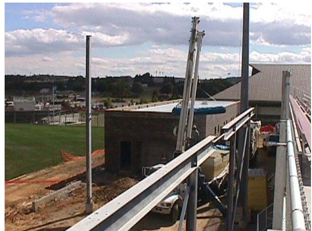
McComas Soccer Field Restroom and Bleacher Construction
