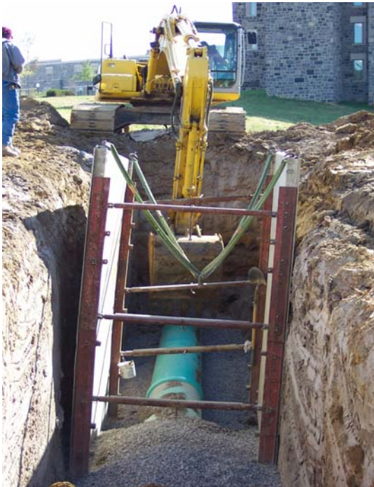
New Sanitary Sewer Project
