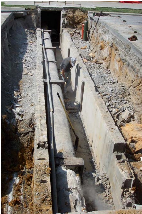
Steam & Water Mains at Washington St. Improvements
