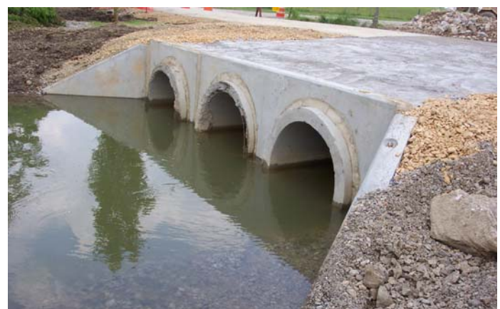
Plantation Road Creek Crossing Improvements
