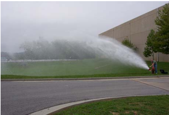
Testing Fire Hydrants
