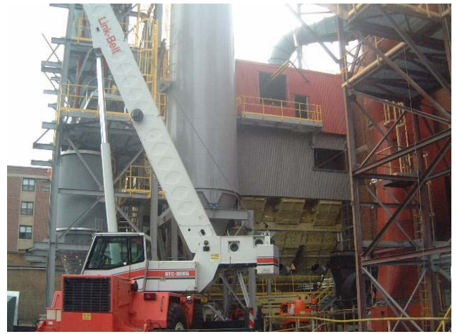
Construction of New Air Pollution Controls
