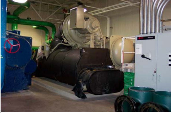
Chilled Water Expansion Project
