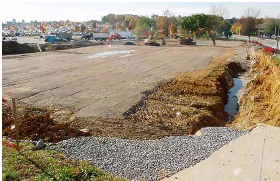
Site Grading for Surge Building
