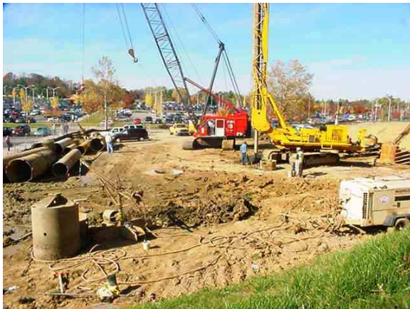
Construction for BC Lab
