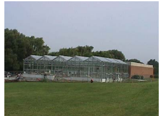
New Greenhouse added to ESL Facility
