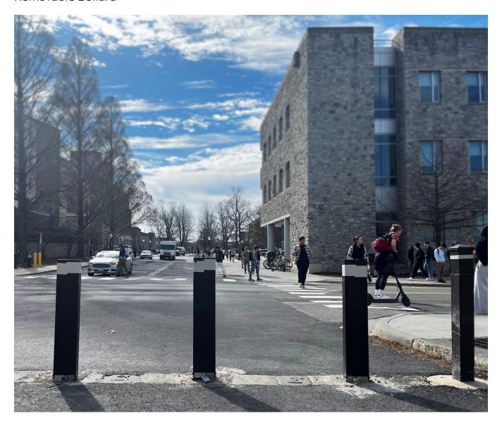
Vendor MaxiForce (Collapsible Bollards - MCSP-SS2-EZ) with heavy duty aluminum inserts
