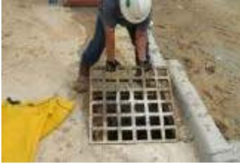
Remove grate from catch basin.
