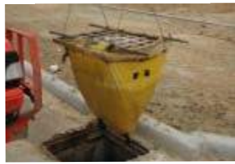
Removed Siltsack® is now ready for cleanout.
