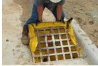
Slide Siltsack® over one side of grate.
