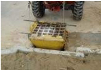
Slowly remove Siltsack® from inlet.
