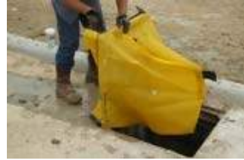
Slide Siltsack® over opposite side of grate.
