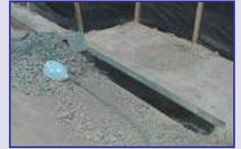
Failed Inlet Protection
