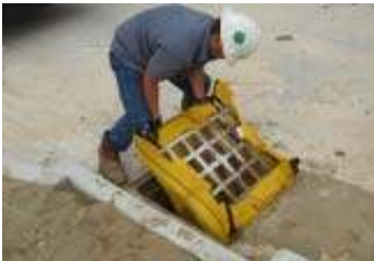
Replace Siltsack® and grate inlet into recess.
