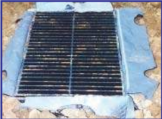
installed Siltsack held in place by grate.
